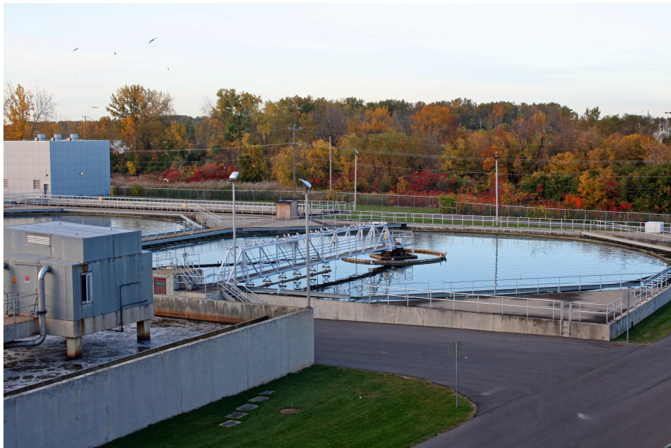
(Metropolitan Waste Water Treatment Facility)
