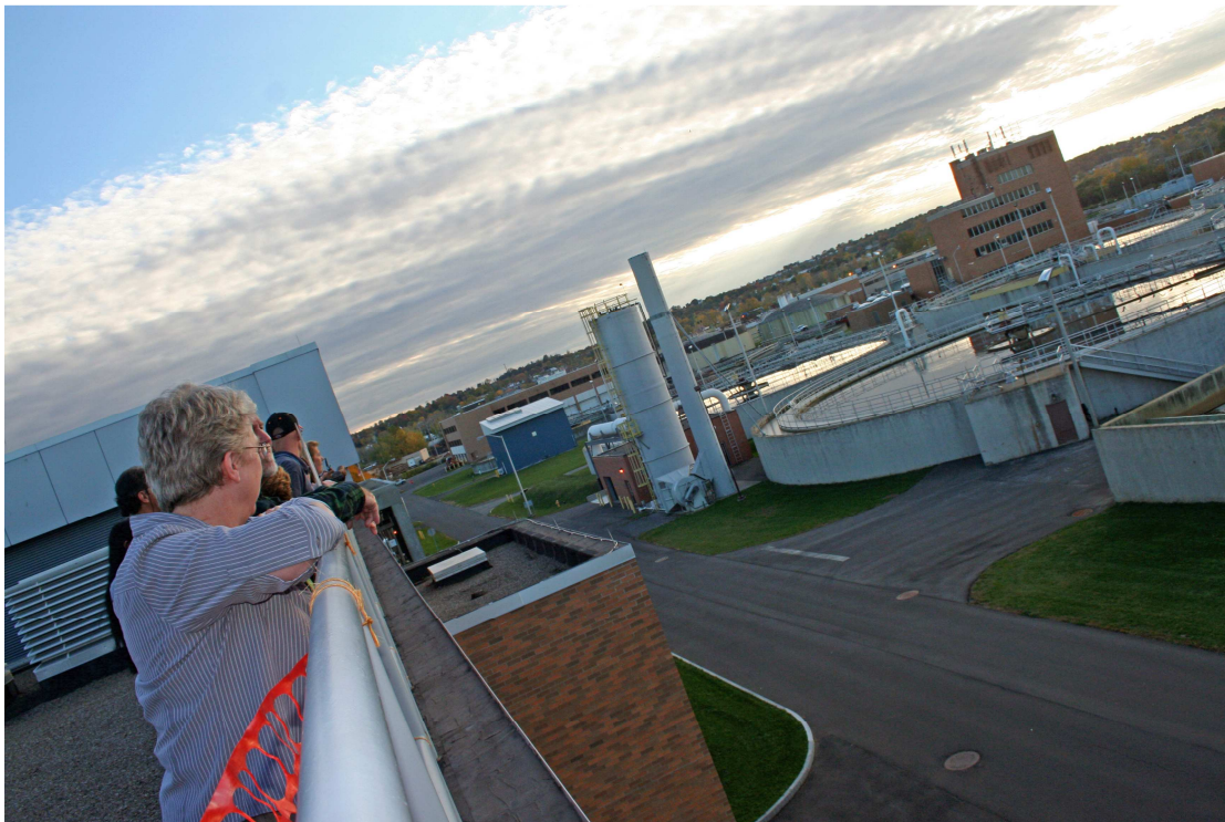
(Metropolitan Waste Water Treatment Facility)
